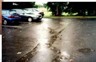
Earlier car park - asphalt with ponding
